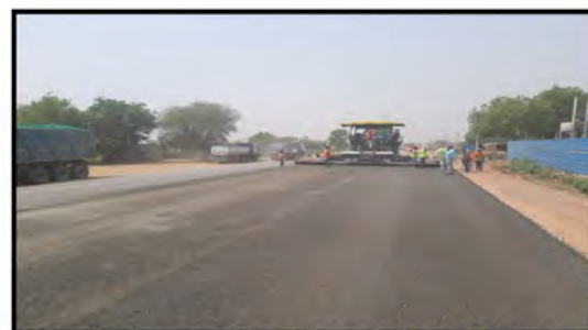
WMM laying in progress from Km 35.410 to Km 35.550 (RHS)
