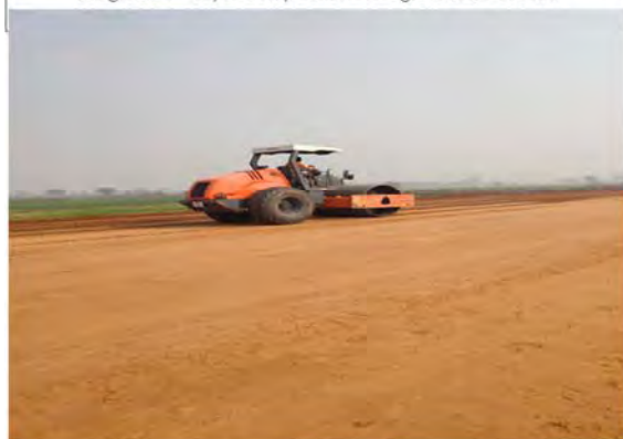
Subgrade Layer Compaction in Progress 25+600 km
