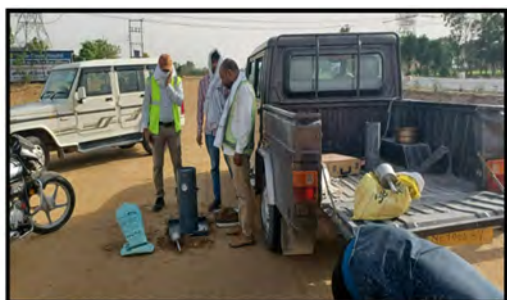
FDD of Embankment Layer km 18.400 to 18.520 Km LHS
