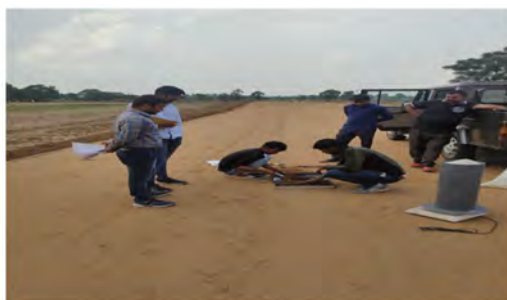
FDD of Embankment 1 st Layer at Ch 20+850 Km
