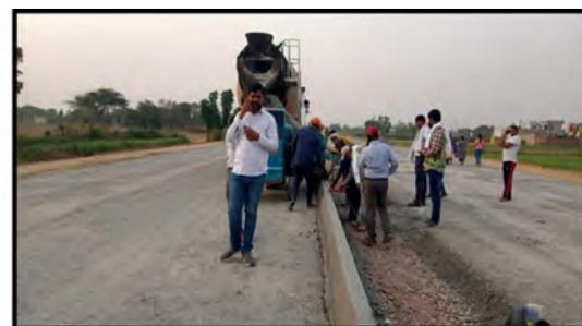
Kerb Laying in progress from Km 21.780 to Km 21.880 (RHS)
