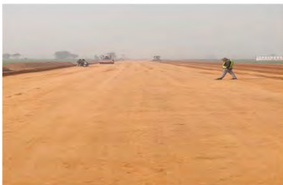
Subgrade 1 st Layer Compaction in Progress at 25+500 Km
