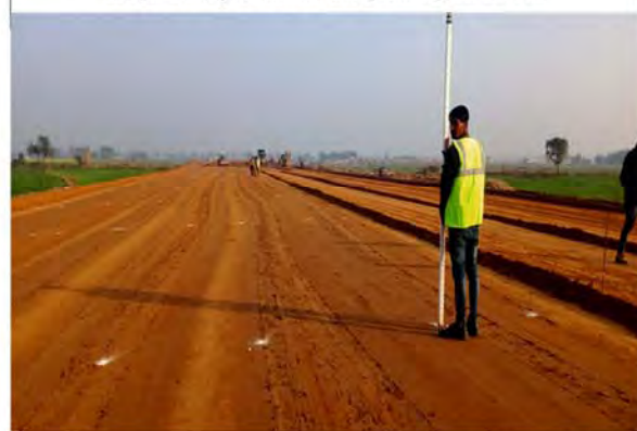
Subgrade Layer Preparation in progress at Ch 25+800 Km
