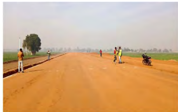
Subgrade Top Level checking in Progress 25+700
