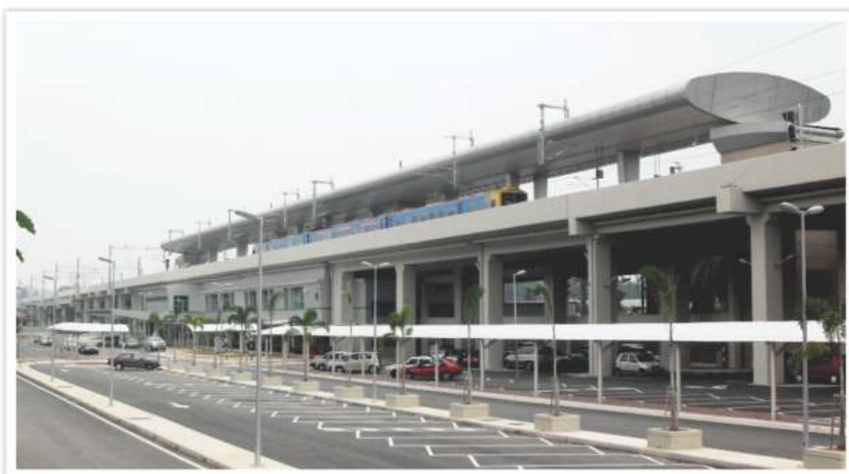
Station Building on Viaduct in Malaysia
