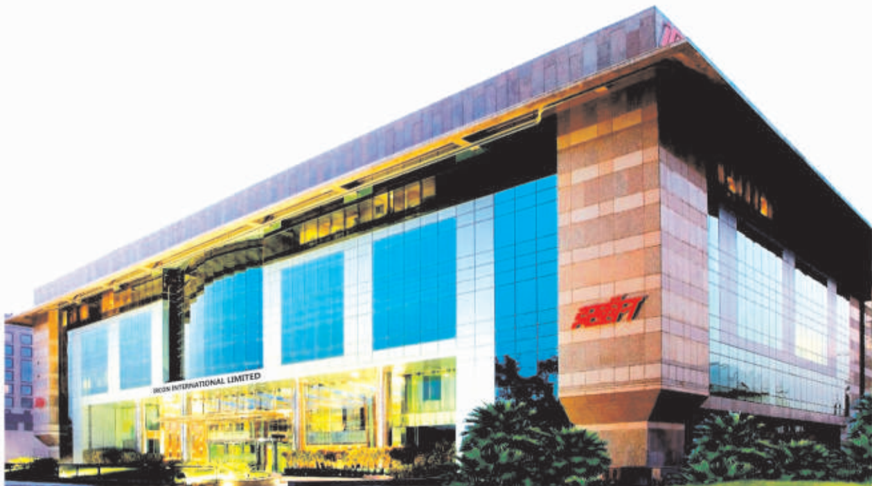
Corporate Office Building of Ircan at Saket, New Delhi
