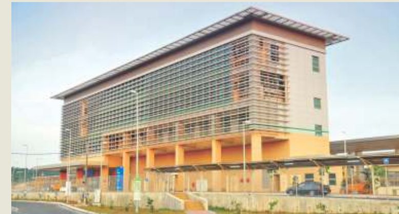
Gemas Station Building of Seremban - Gemas Electrical Double Track Project, Malaysia
