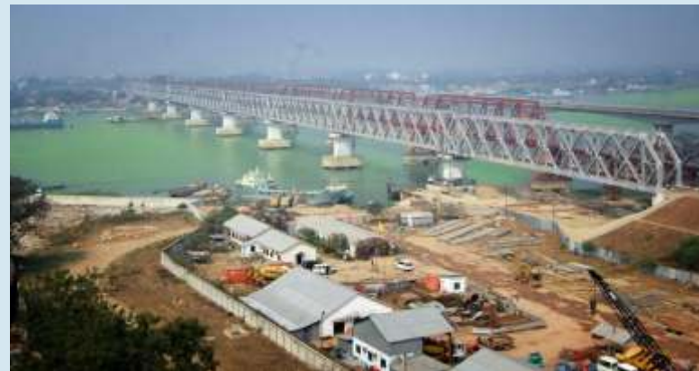
2nd Bhairab Bridge Bangladesh
